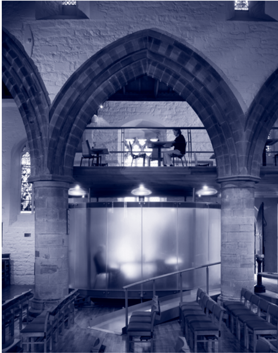
Mezzanine eating area in All Saints' 1997 award-winning conversion, with Tardis-like vestry beneath (photo courtesy Martine Hamilton Knight / Builtvision)
