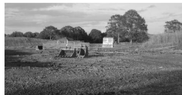
Works progressing well at the Enterprise Zone
